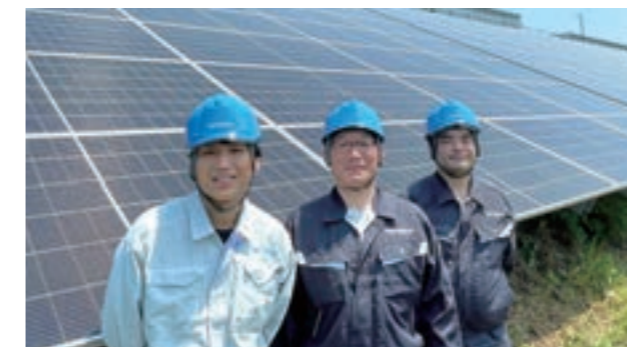
Newly installed solar panels at Sendai Works
