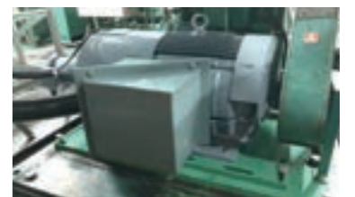
Installed take-up inverter motor
