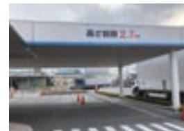
Measures to prevent collisions by indicating height limits
